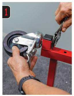
Install (4) **Total-Lock Caster Wheels** into **Side Frame** as shown.
